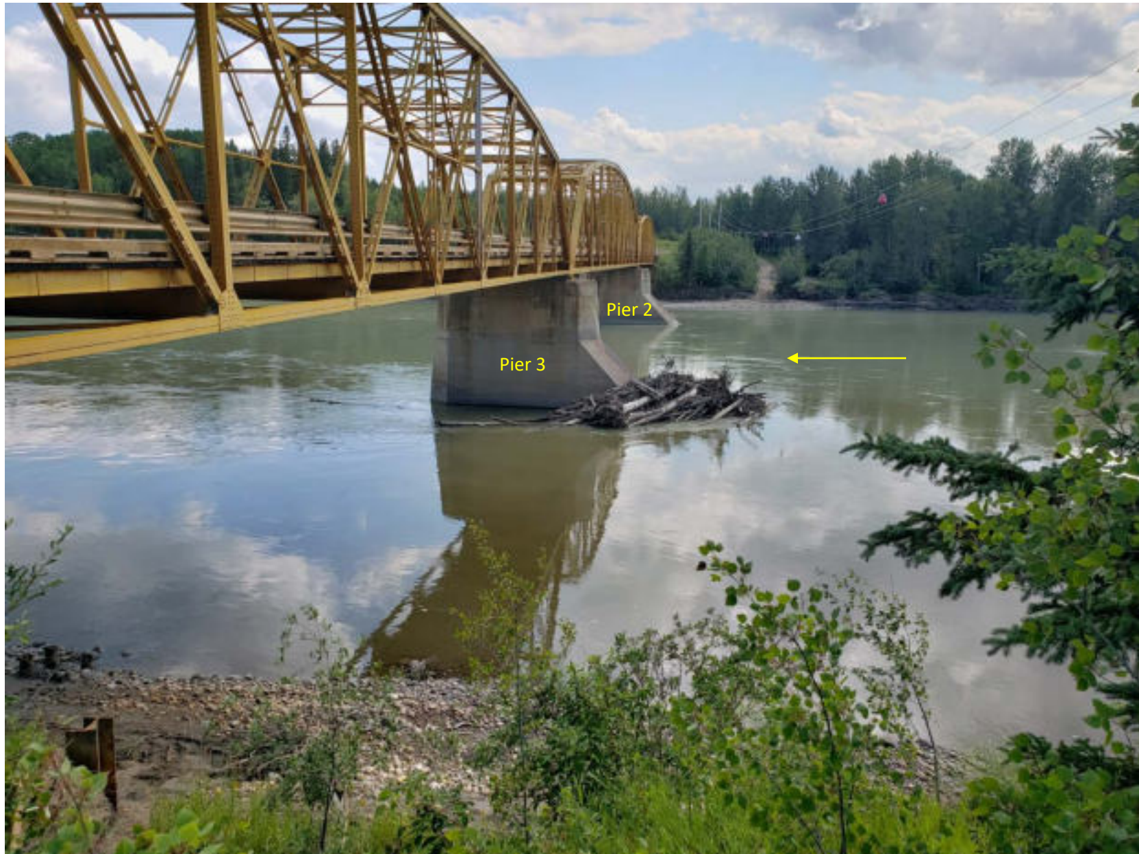
Site Photo 1 – upstream face of the bridge
