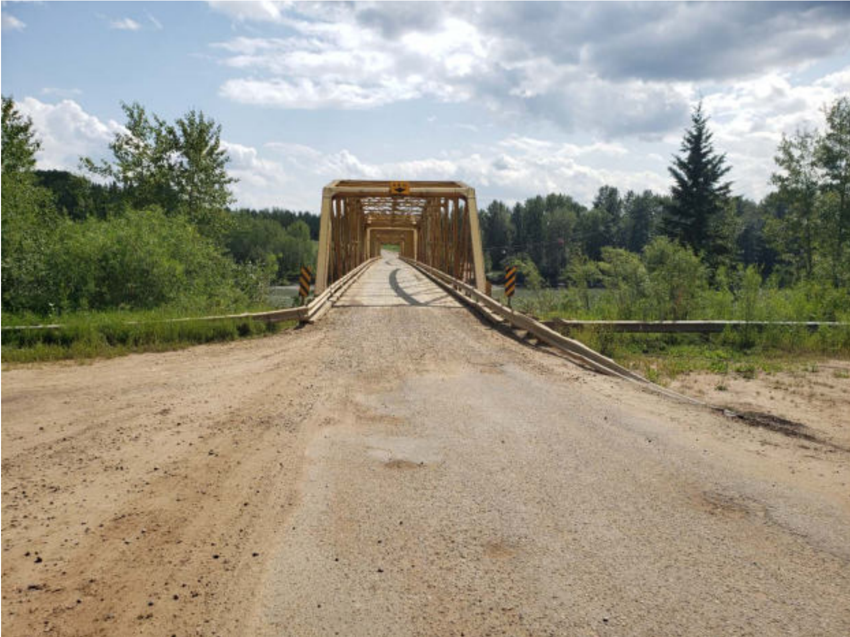
Site Photo 8 – looking south
