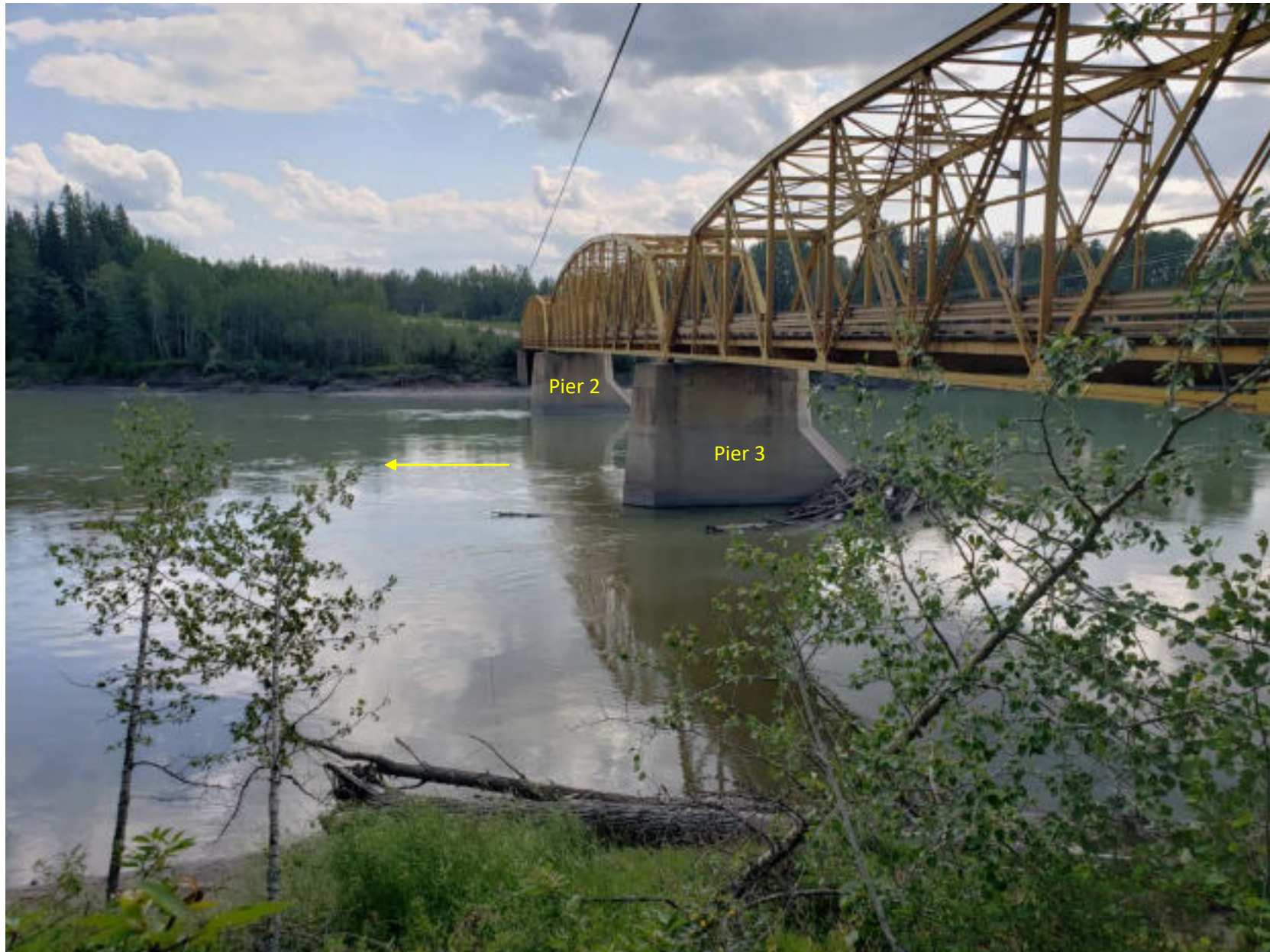
Site Photo 2 – downstream face of the bridge
