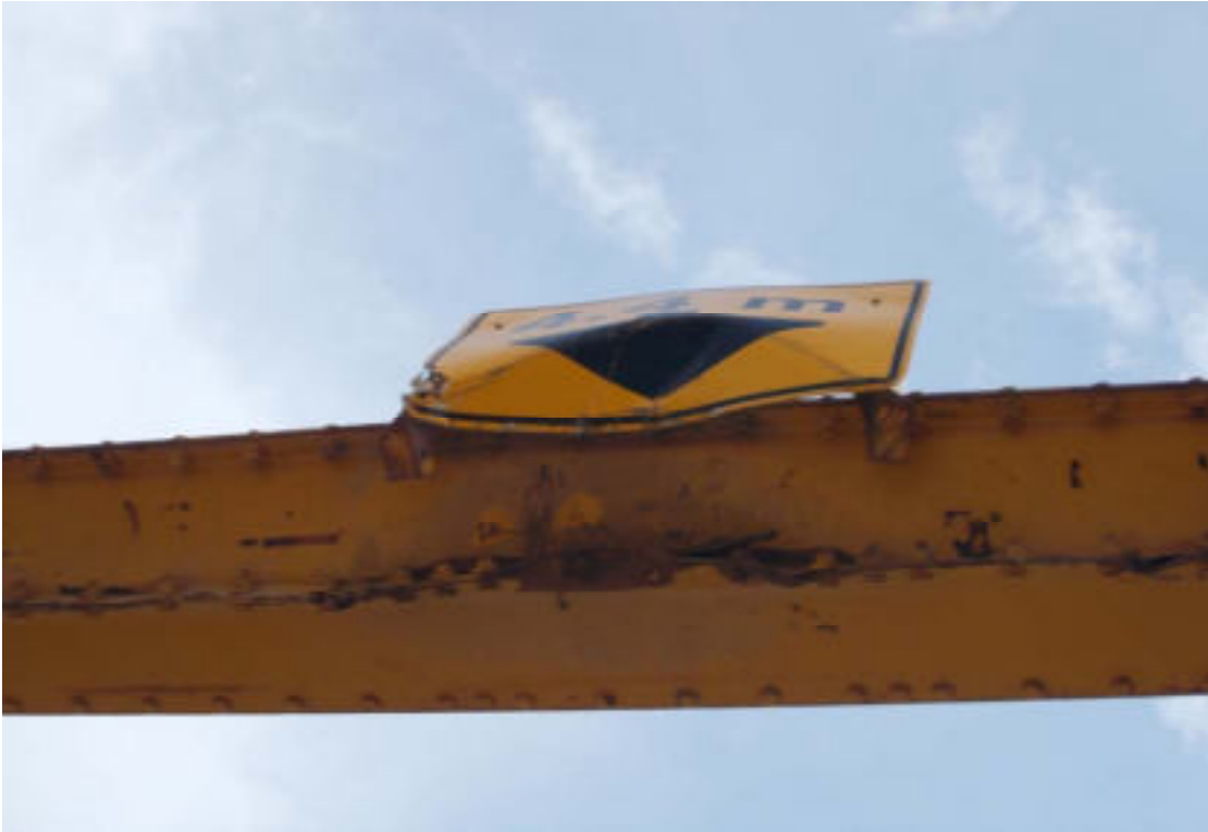
7. Vertical clearance sign and S6 north portal were damaged
