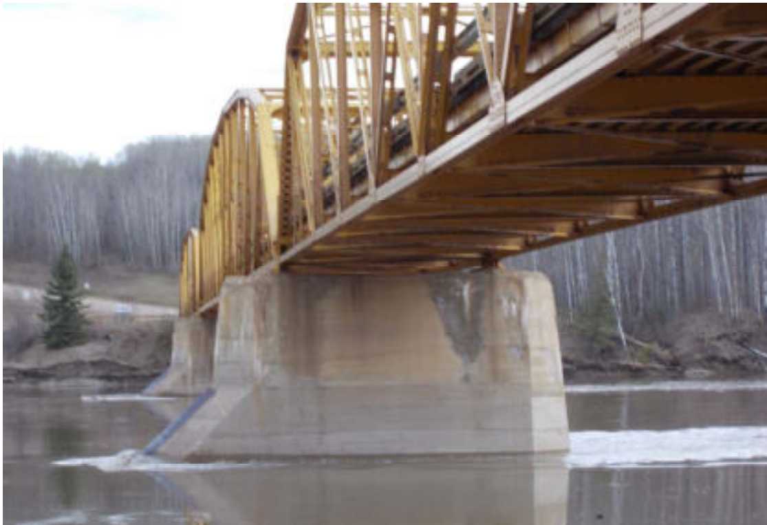
49. Erosion around Pier 3
