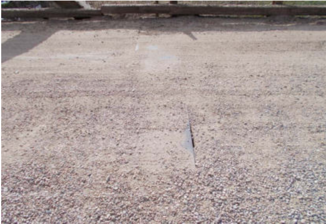
19. Steel coverplate at Pier 6 joint
