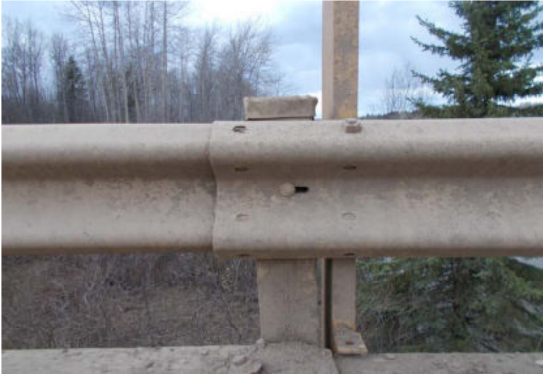
25. 7 splice bolts at S3 NW
