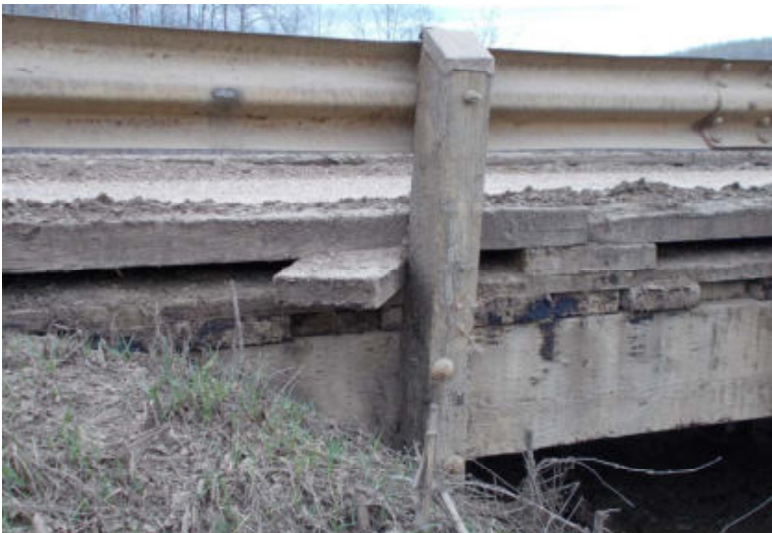
21. S3 one WG at west side was damaged
