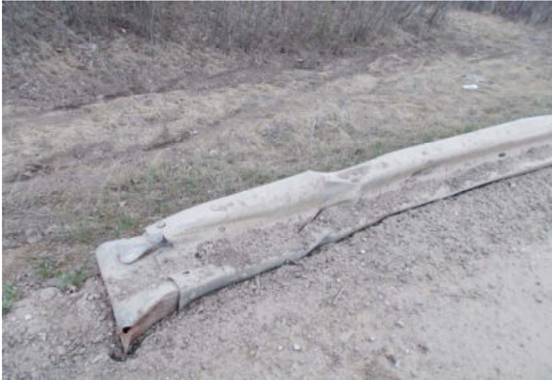
11. SW TD was damaged
