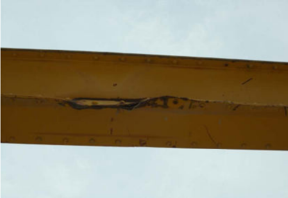
31. SP6 south portal was damaged
