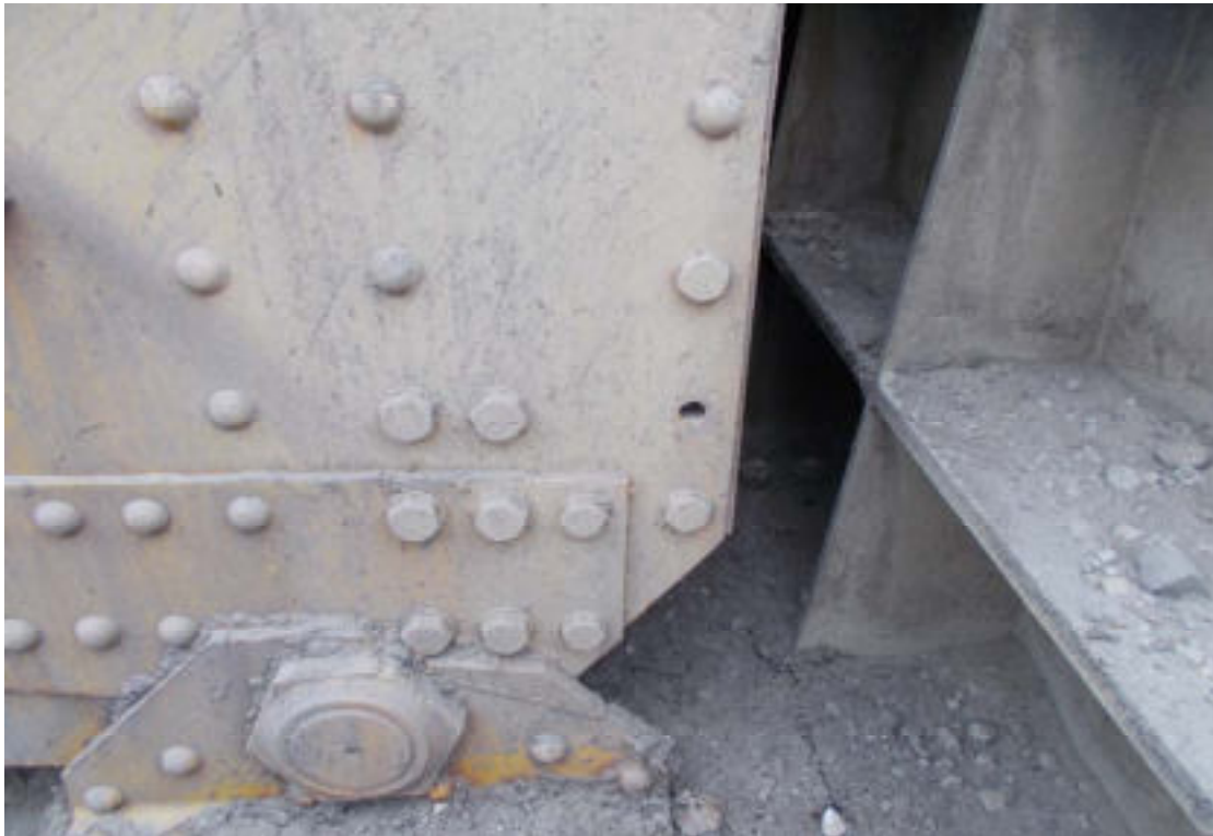
35. One bolt missing at SP6 gusset plate near bearing
