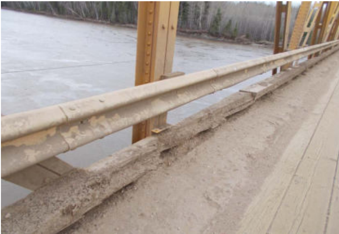
23. S5 one WG was damaged at east side
