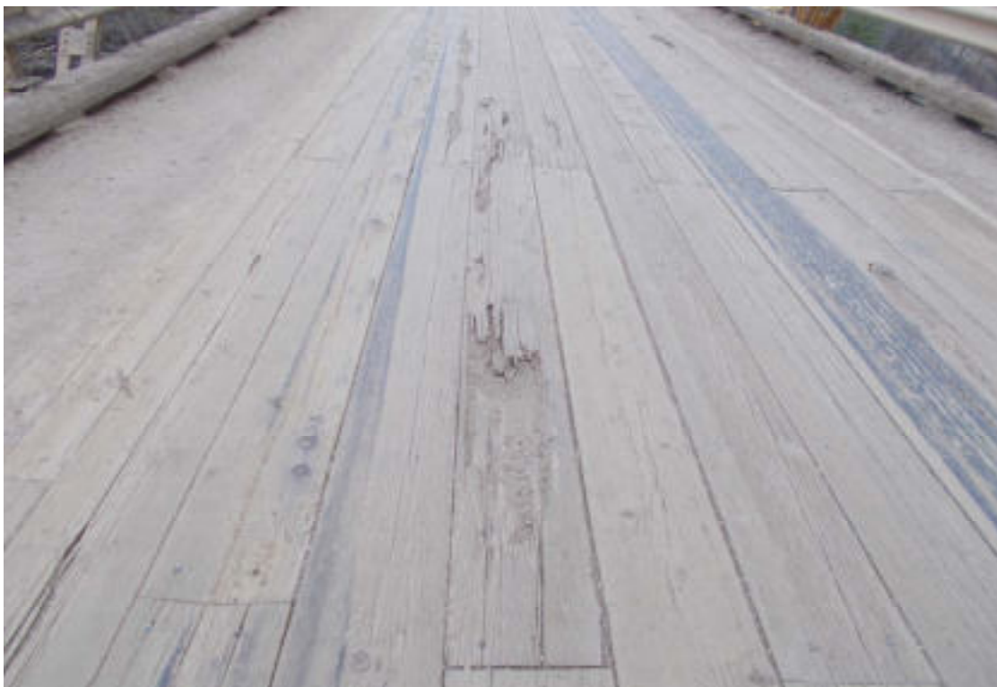
15. Rotten deck planks at SP3
