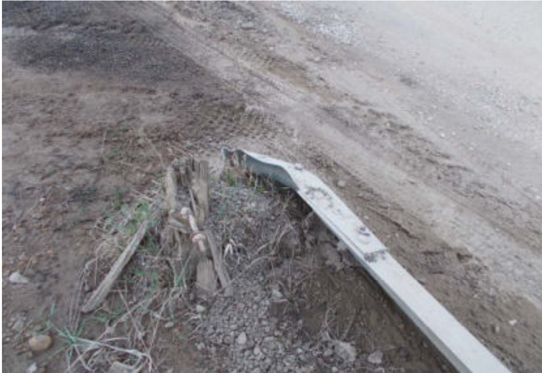
9. SE TD end disconnected from post and post broken
