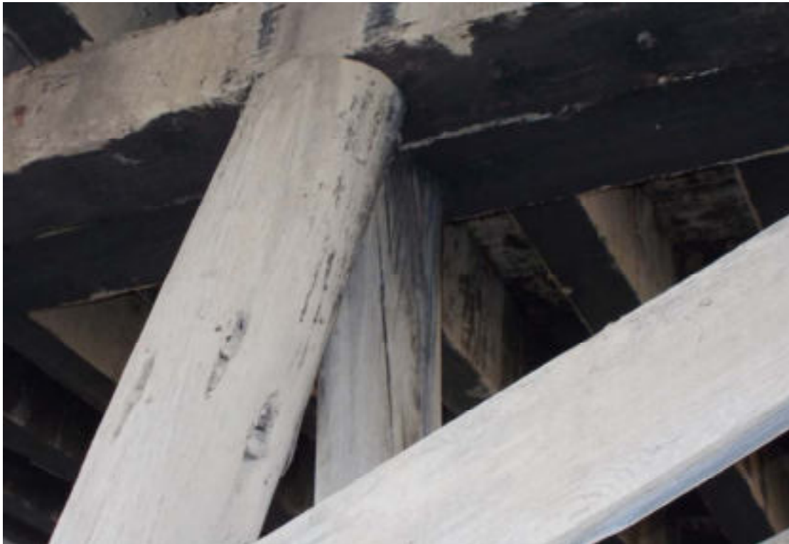
47. Wide checks at Pier 2 timber piles - typical
