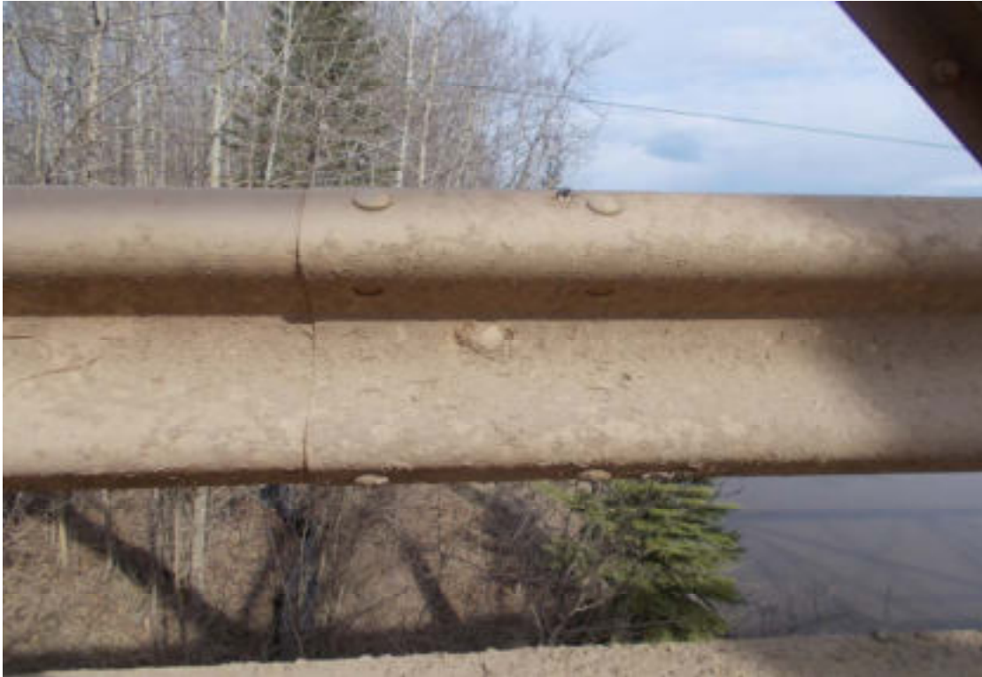
27.4 splice bolts missing at SP6 east side - typical at multiple locations
