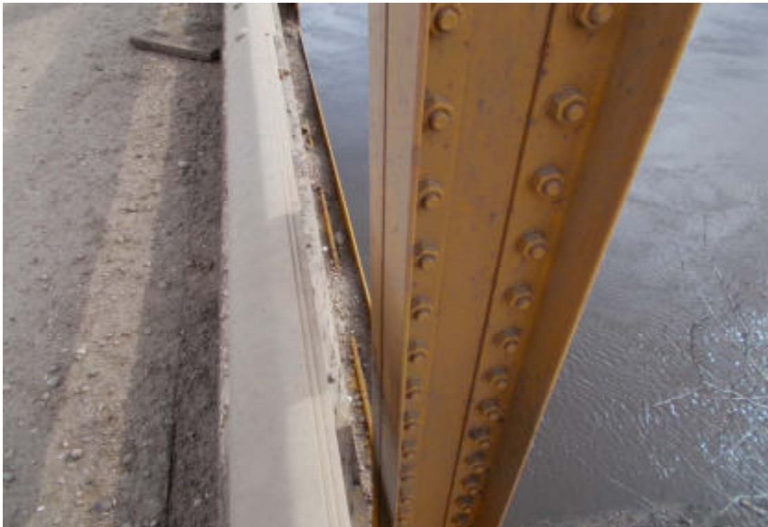
25. 7 splice bolts at S3 NW
