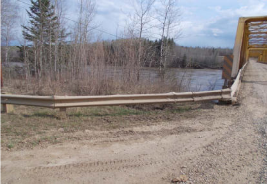
13. 3 posts missing at NE corner
