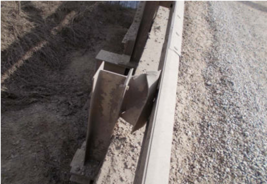
27.4 splice bolts missing at SP6 east side - typical at multiple locations
