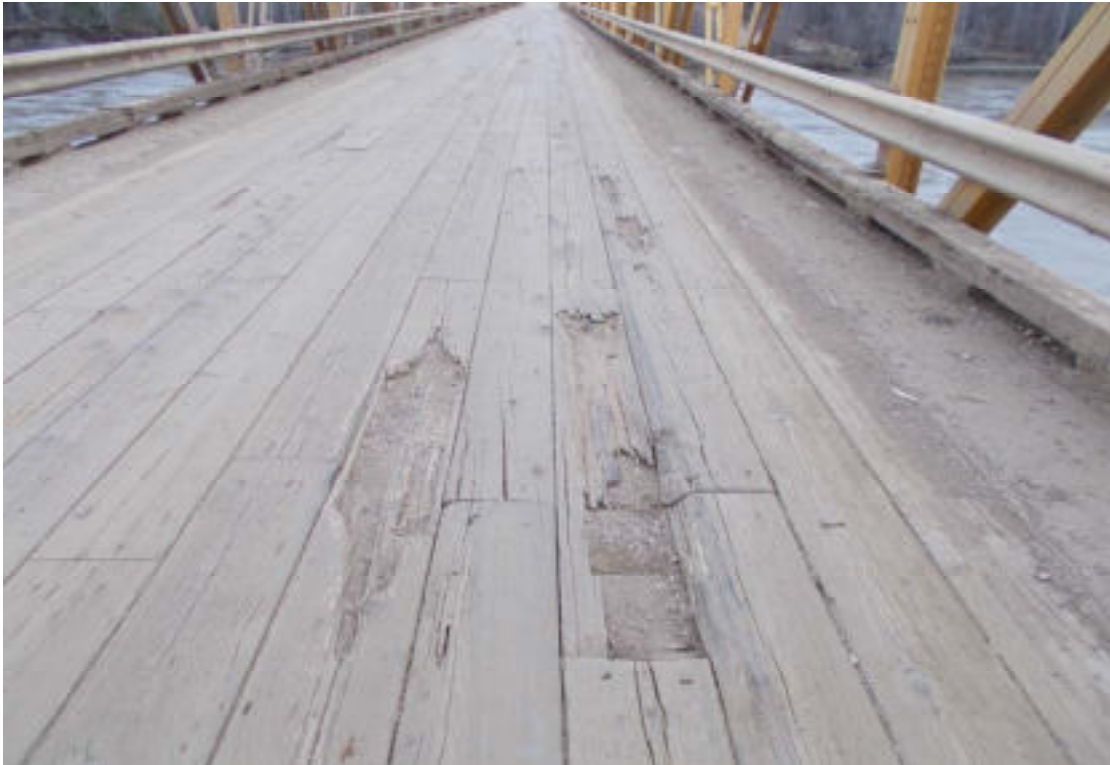
17. Rotten deck planks at SP5
