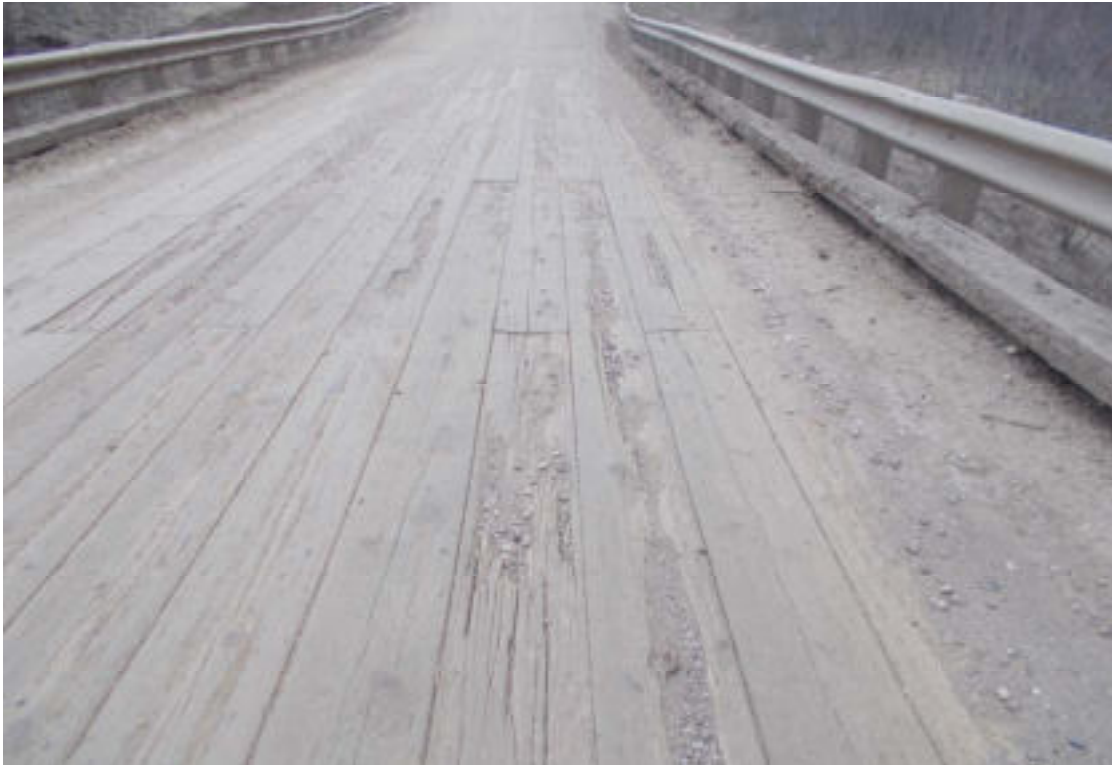
15. Rotten deck planks at SP3
