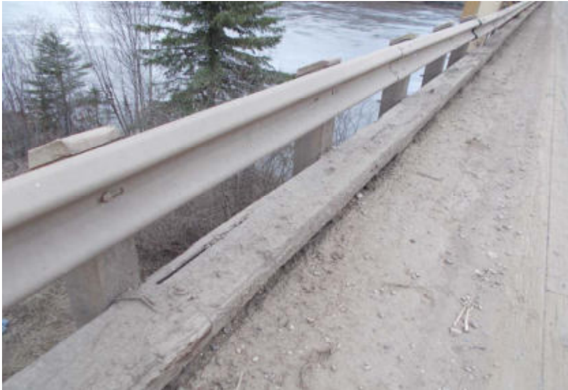
21. S3 one WG at west side was damaged
