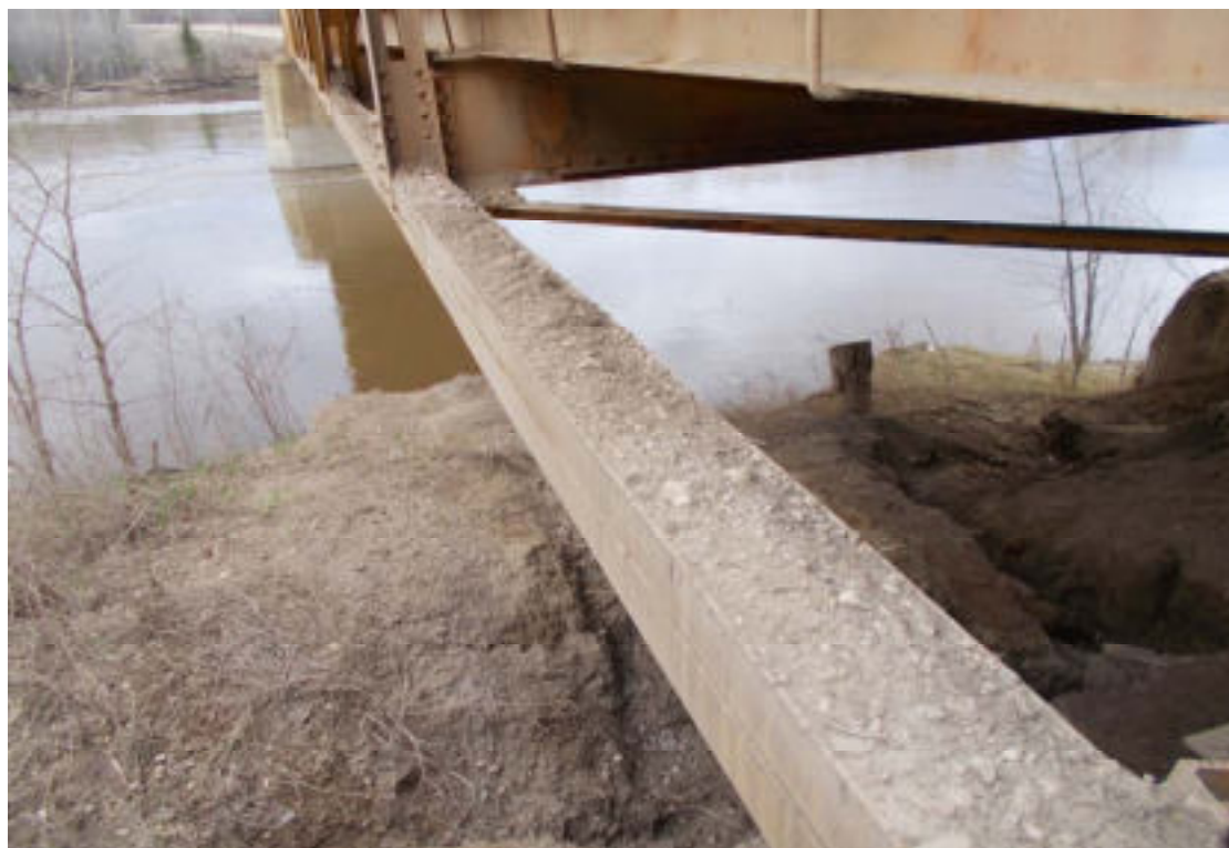
35. One bolt missing at SP6 gusset plate near bearing
