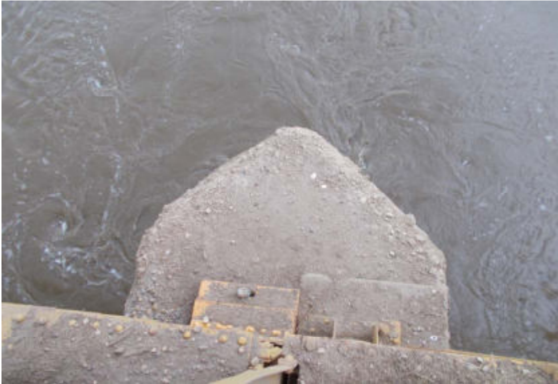
53. P4 east top with heavy scaling
