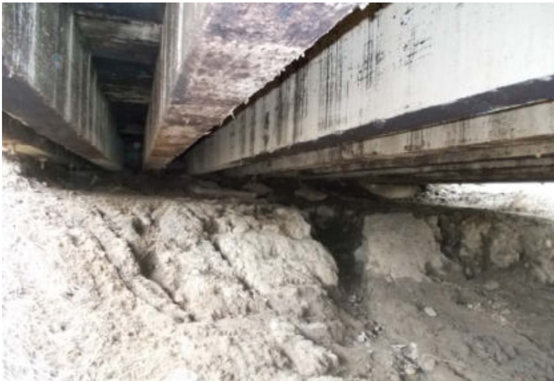
39. SP1 Stringer 11 (left side) bearing approx 95mm on Pier 1
