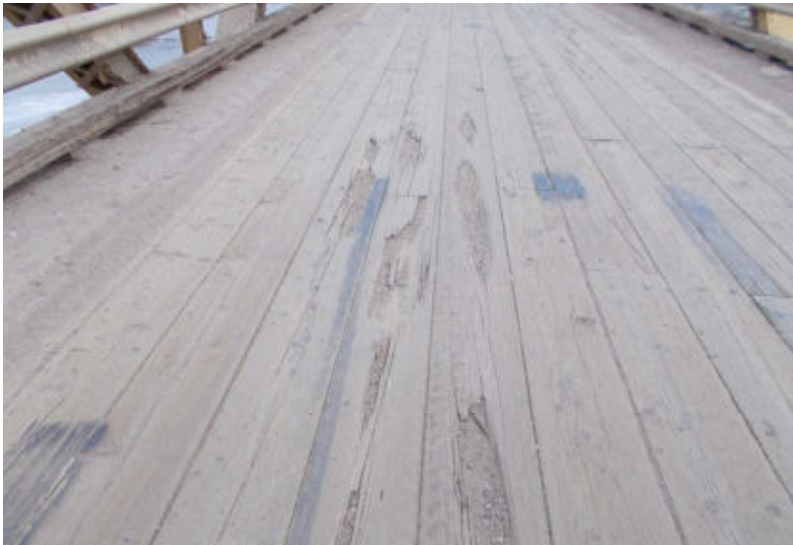
17. Rotten deck planks at SP5
