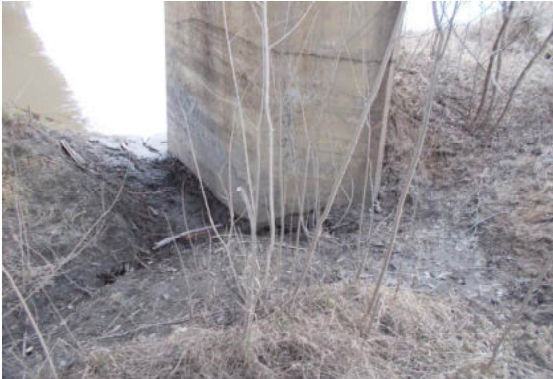
49. Erosion around Pier 3
