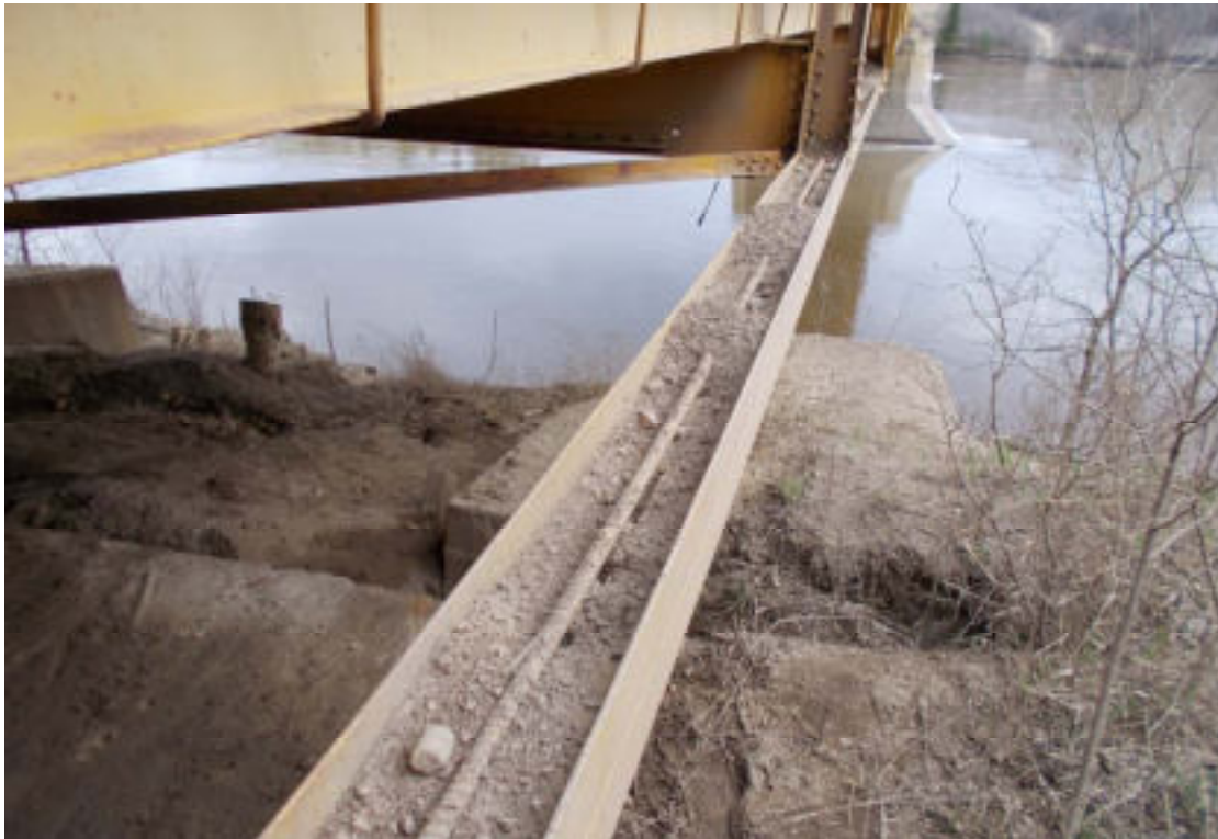
33. Dywidag bar at SP6 west bottom chord. Dirt on bottom chord
