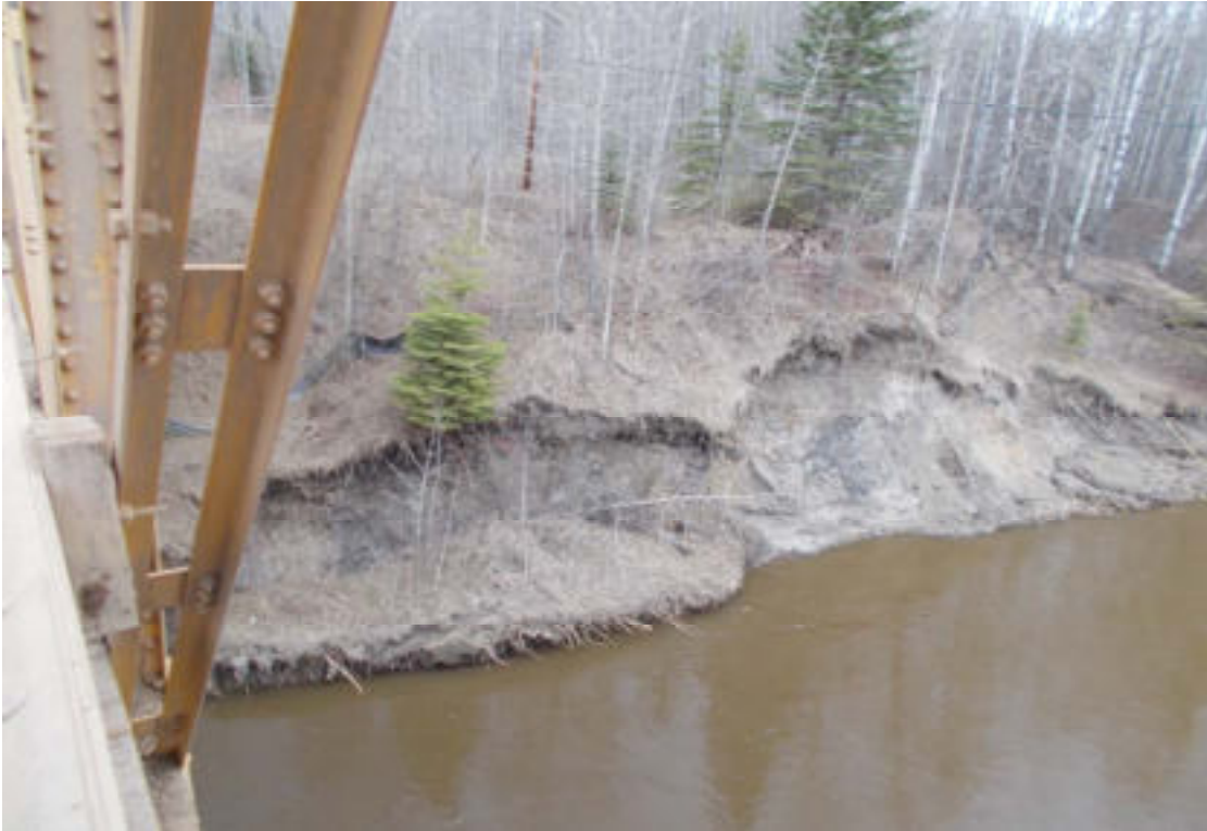
55. NE hill is sloughing
