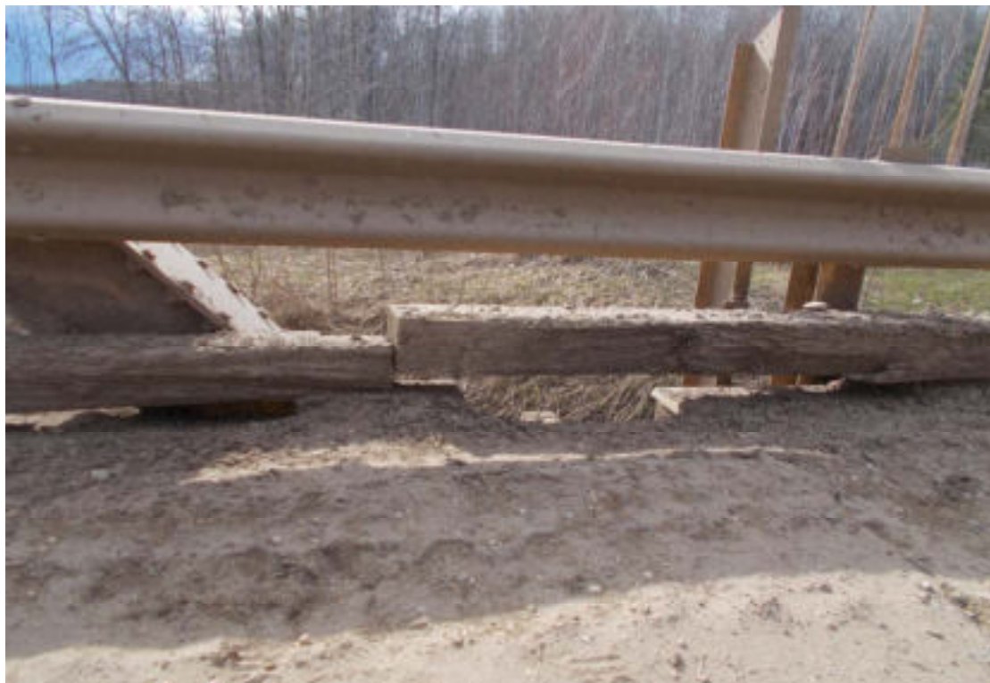
23. S5 one WG was damaged at east side
