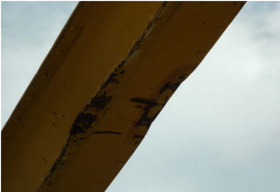
29. 3mm long crack was marked on SP4 U7L6E near U7
