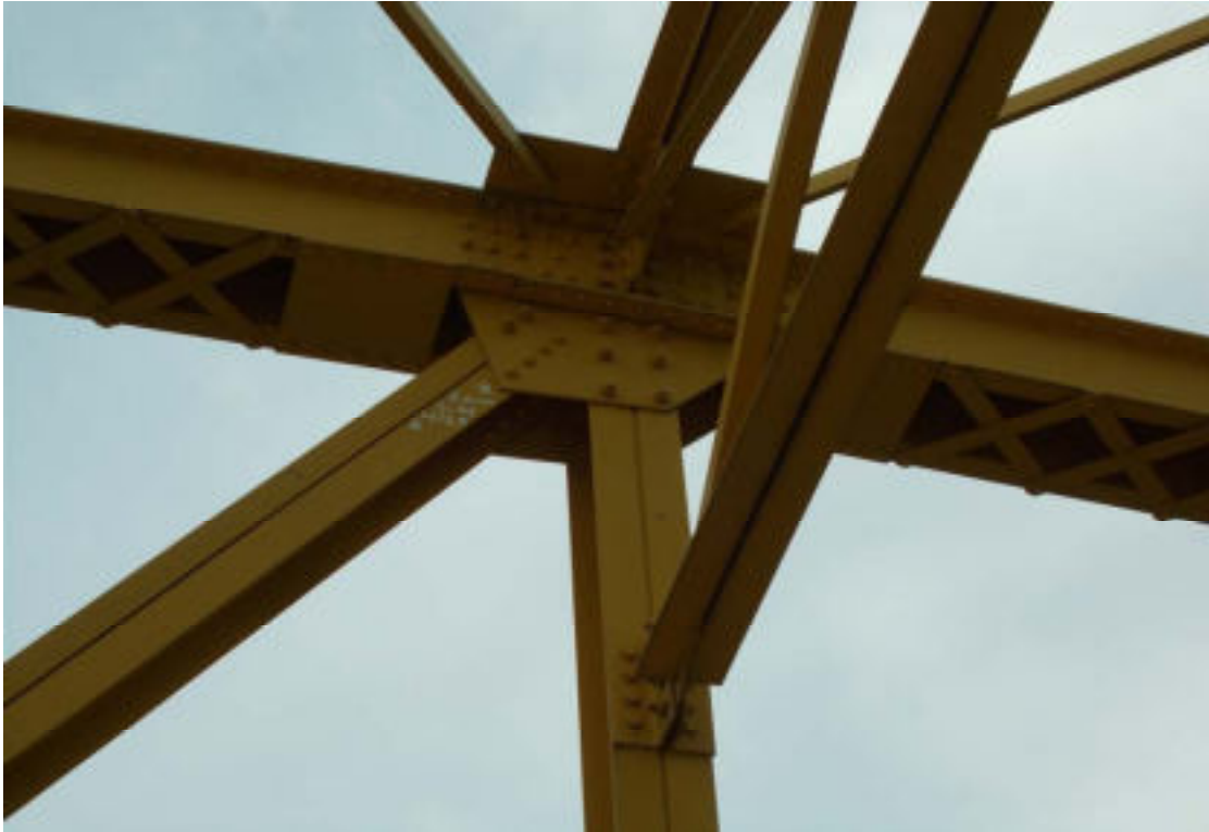
29. 3mm long crack was marked on SP4 U7L6E near U7
