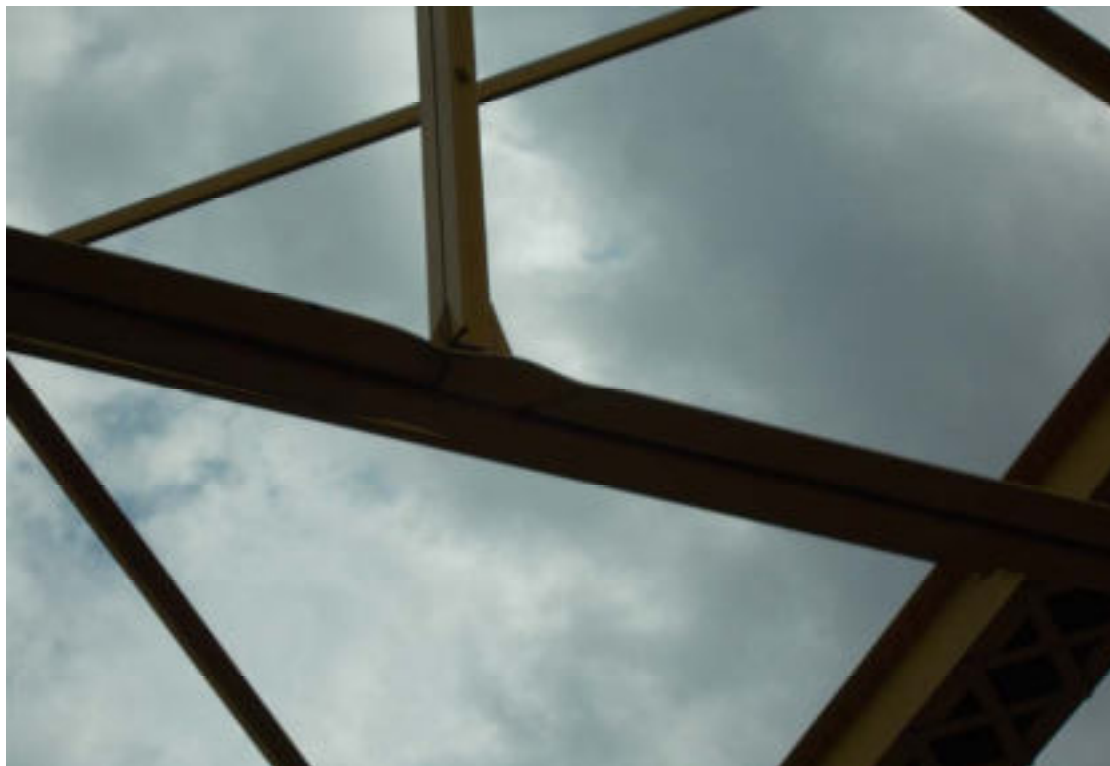
31. SP6 south portal was damaged
