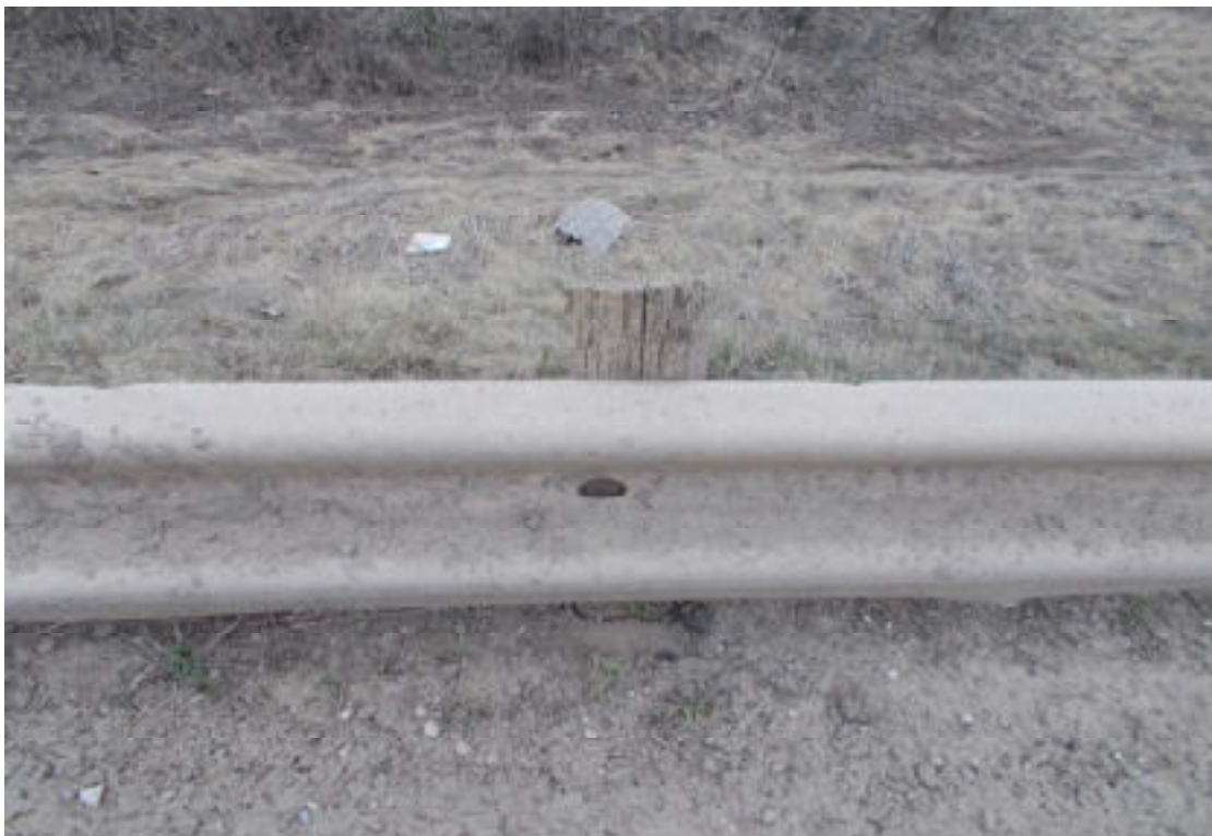
9. SE TD end disconnected from post and post broken
