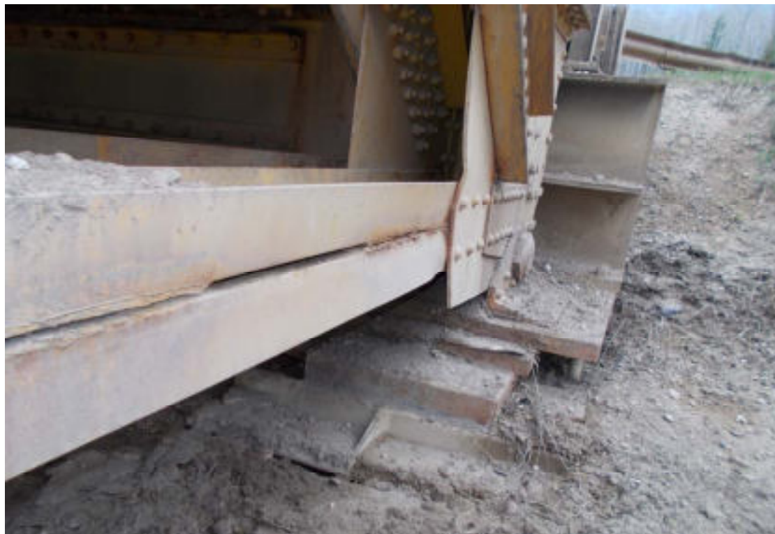
33. Dywidag bar at SP6 west bottom chord. Dirt on bottom chord
