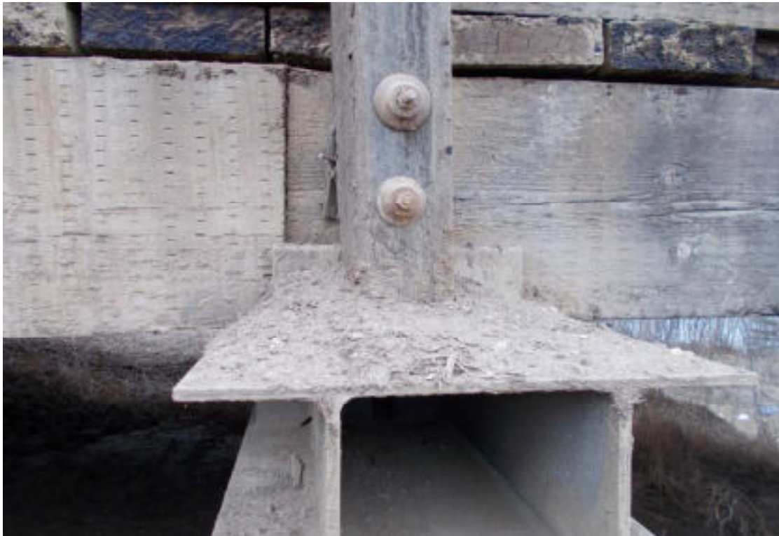
39. SP1 Stringer 11 (left side) bearing approx 95mm on Pier 1
