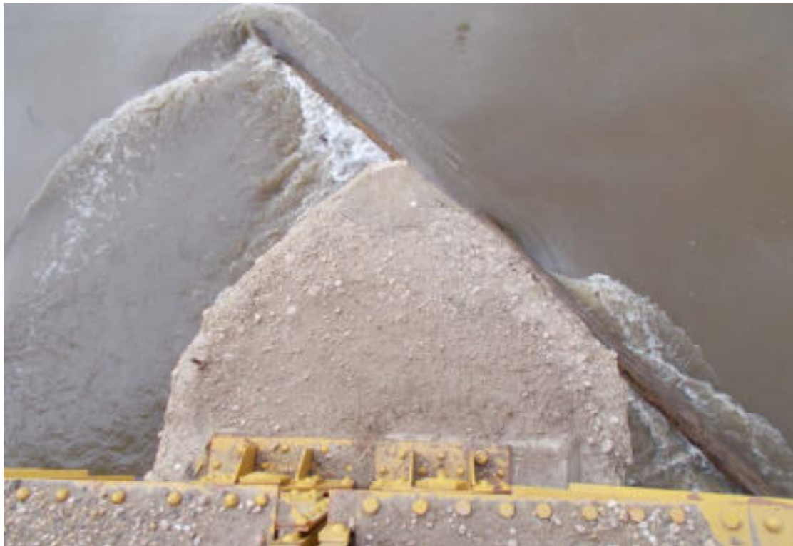
53. P4 east top with heavy scaling
