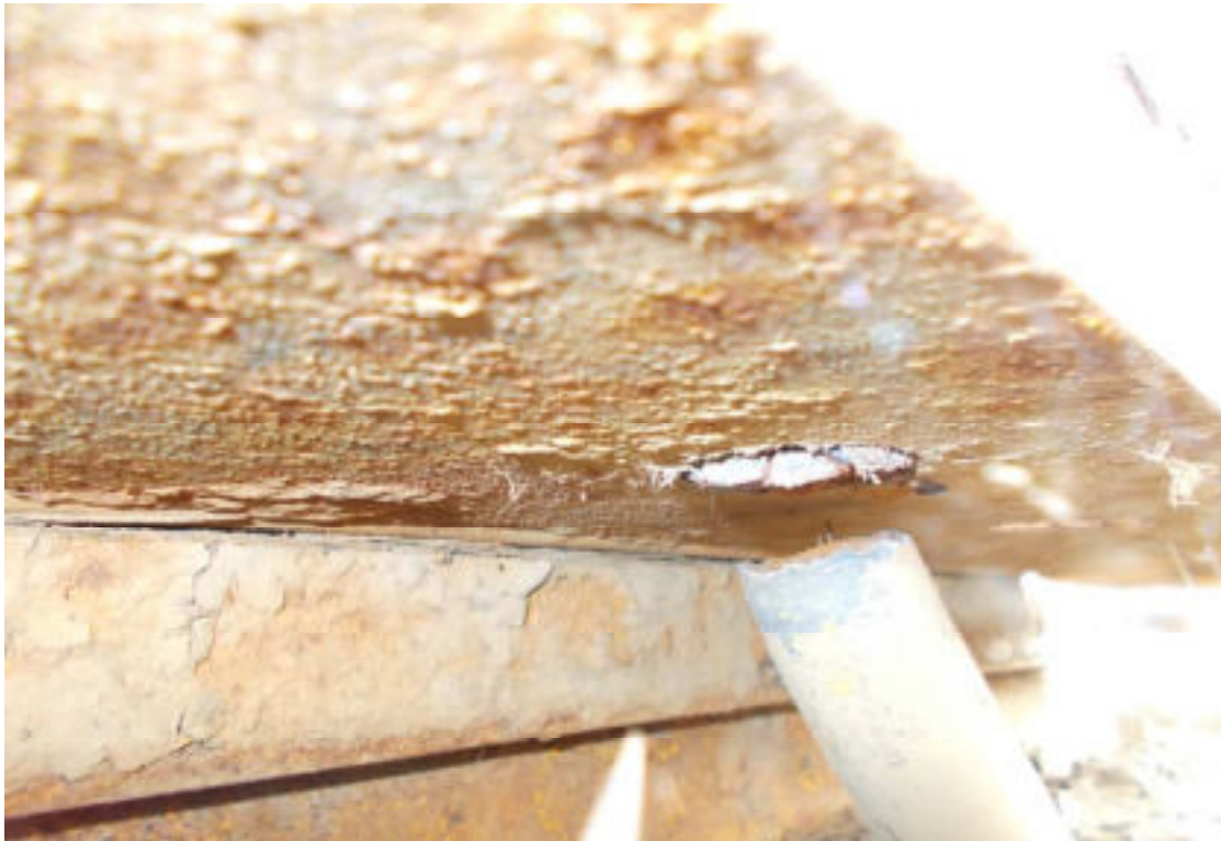
37. One bearing A/B at P6 west bearing sheared off
